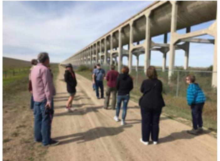
Christina leading the Walking Tour of the Brooks Aqueduct
